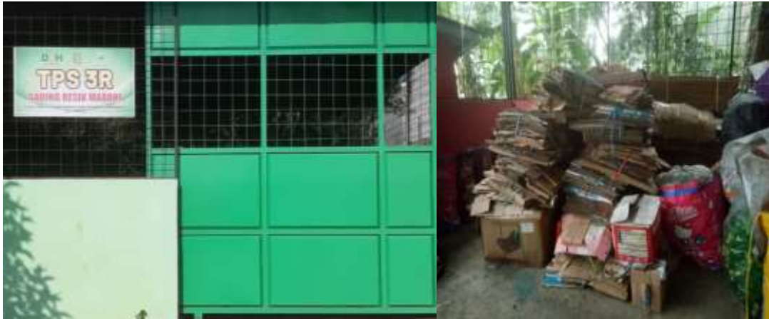
Picture 4. TPS3R Building Gading Resik Madani; Generation of Non-Organic Waste with Post-Sorting Value
