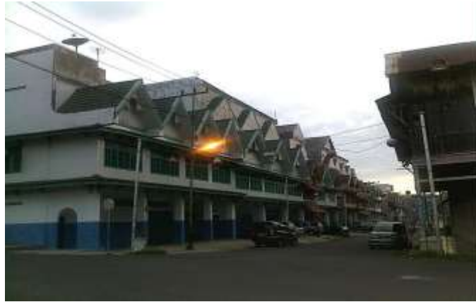
Figure 2: Bengkulu Chinese Shophouse 2007 Source: Simpang Limo, 2011
