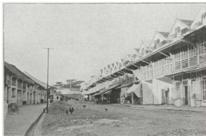
Figure 7: The result of the 1917 renovation of the Chinese shop house in Malabero, Bencoelen.
